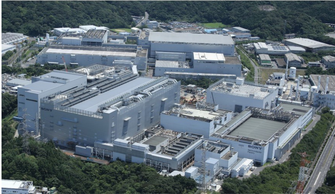
SCK Nagasaki Technology Center
